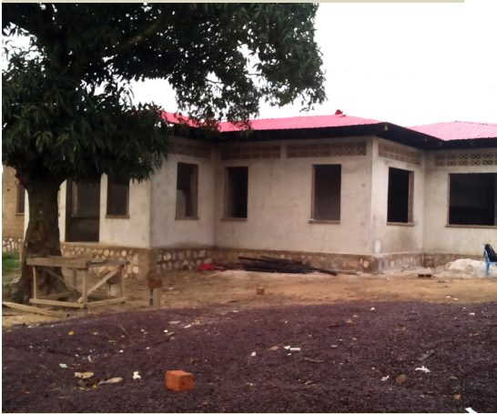
The new hospital building at SD DR Congo's "Mother and Child Hospital at Kwilu Ngongo
