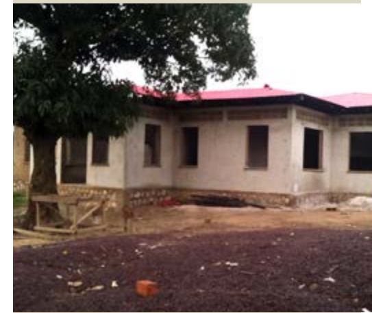
The new hospital building at SD DR Congo’s “Mother and Child Hospital at Kwilu Ngongo
